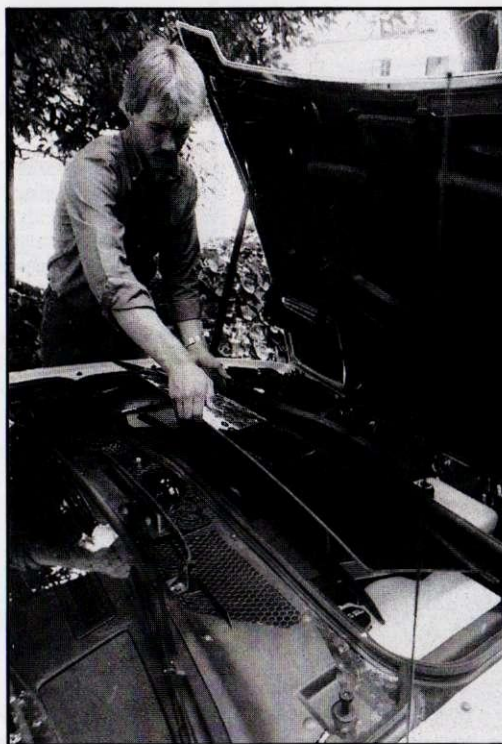
Removable glass panel for optional sunroof stores in Fiero's forward compartment.
